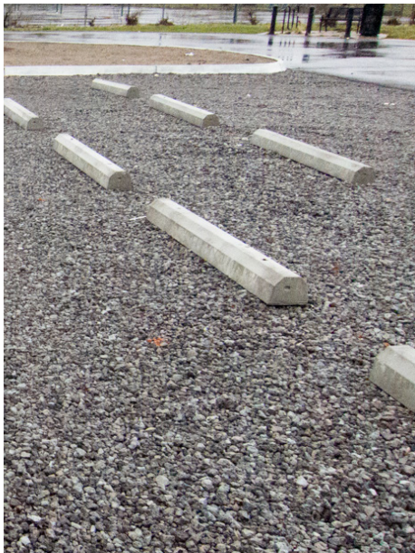
Three examples of DWSD's sustainability efforts in stormwater management as seen through the bioretention gardens at (l-r) the Crowell Recreation Center, Oakdale Boulevard and an example of a permeable lot at Stoepel Park.
