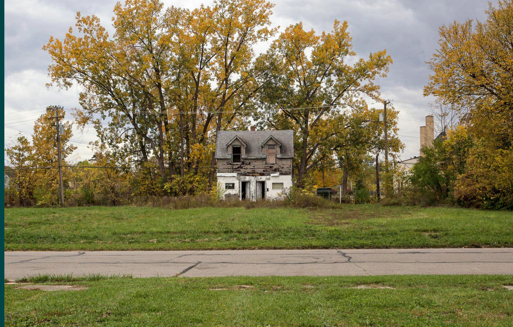
An abandoned home sits between two vacant lots during Detroit’s housing crisis. Major banks approved just 375 mortgages in Detroit in 2013.
